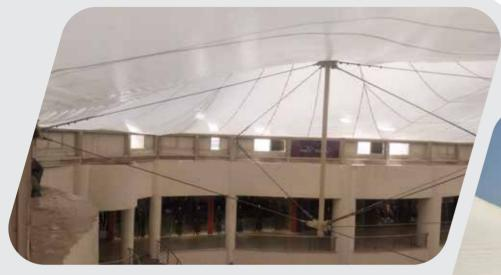
• 1200 m<sup>2</sup> of Tensile membrane structure
